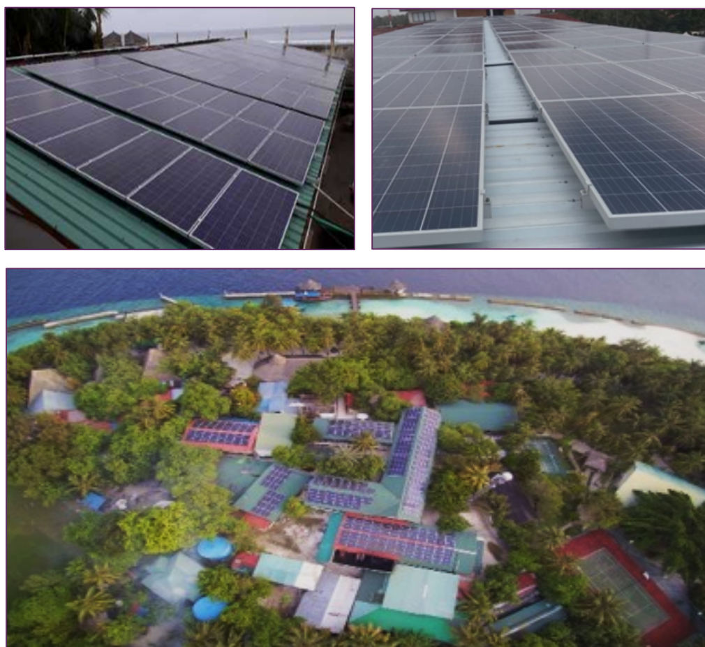
Solar PV Systems at Cinnamon Dhonveli Maldives, Hikka Tranz by Cinnamon and Ellaidhoo Maldives by Cinnamon
